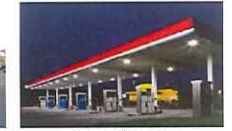
Station de service
